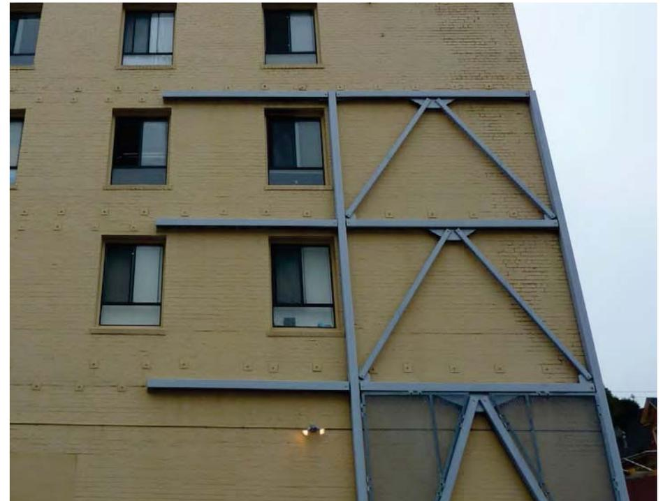
Example of seismic retrofit of masonry wall
